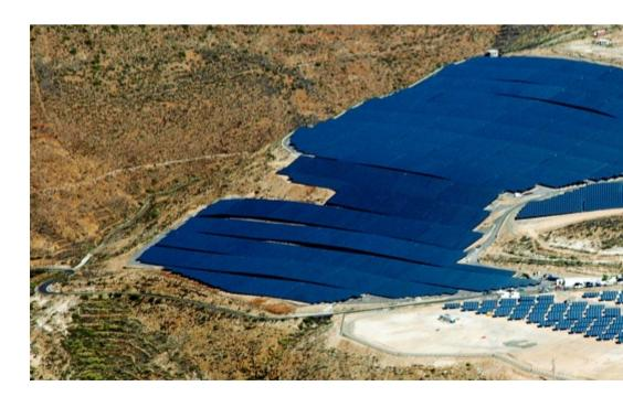
The power plant is the first stage of a project of 5 MW. This first stage was installed in the second half of 2008. The 1,4 MW remaining is still to be installed to complete the total power. It is a mid voltage installation with connection to the grid located in the 204 plot of the area 7 of the Municipal Term of Arico in a place known as "Las Esquinas".
