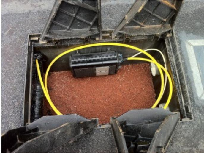
IT<sup>3</sup>'s network passes through underground conduits in both road and rail infrastructures. It consists of an estimated 200 kilometres ring network with a maximum capacity of 504 fibre optics (all segments fully redundant).
