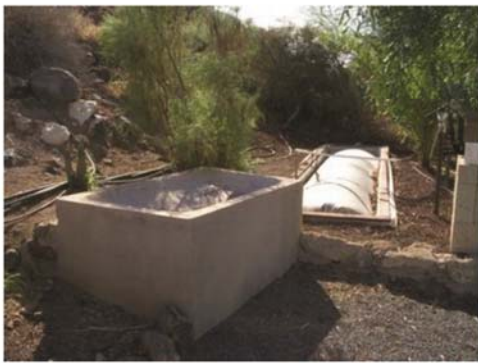
Methane Biogas digester
